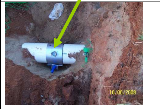
ⓘ2 4.3 & 4.7 No 3 fitting and Meter union
