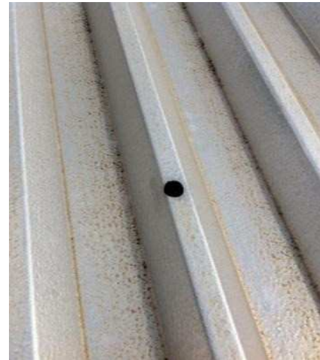
Figure 5-2: Holes (Missing Bolts) in Roof of Pine St (Potable) Reservoir
