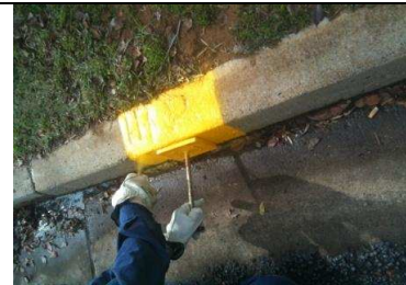
□6 Step 4.3,4.4 Paint gutter using protective cover
