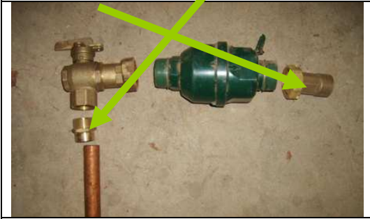
ⓘ3 4.4 & 4.8 Ferrule bend and No 2 Fitting
