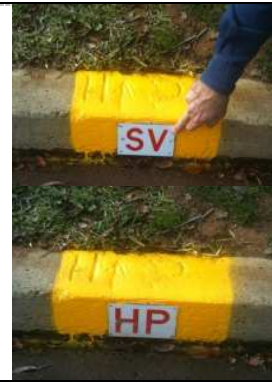
□6 Step 4.3,4.4 Paint gutter using protective cover
