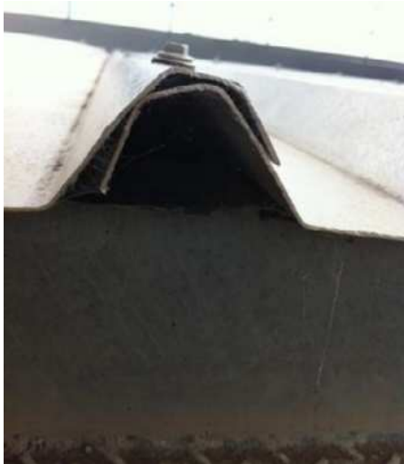
Figure 5-1: Corrugations in Roof of Pine St (Potable) Reservoir
