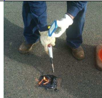
□8 Step 5.3 Tar patch, flame present
