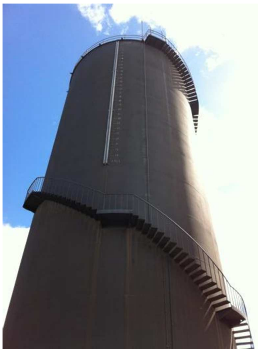
Figure 3-5: Pine St Reservoir (Potable)
