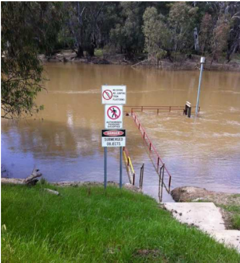
Figure 3-2: Murrumbidgee River Intake (Leonard Street Pump Station)
