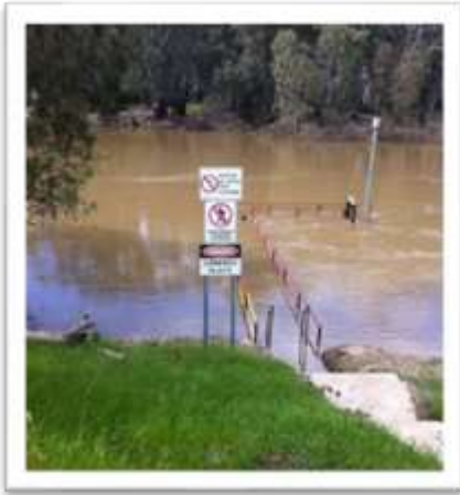
Figure 17: Murrumbidgee River off-take (Leonard Street Pump Station)
