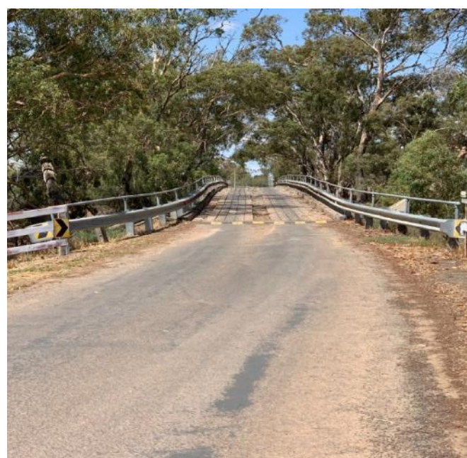
Images (above): Constraint 17.8 Hay - Chainage 6.5km Matthews Bridge over the Murrumbidgee River at Maude 3.8m wide (Timber Bridge built 1967)
