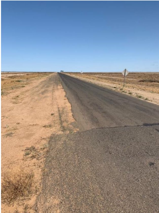
Image (Above) Constraint 25. 5 Hay - Chainage 28.6km to 84.6km– Narrow road from 8m to 6m
