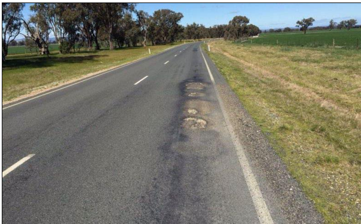
Image (above): Constraint 20.1 Federation - Kywong Howlong Road – inadequate pavement strength. Image from Federation Council
