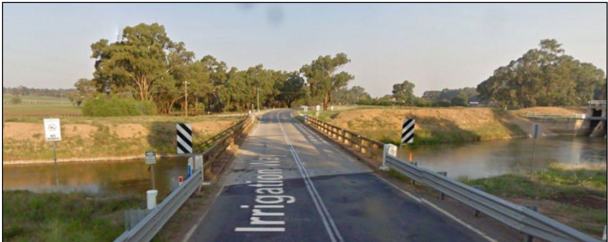
Image (above): Constraint 7.10 Narrandera - Narrow bridge on curve on MR80. Image from Google Street view
