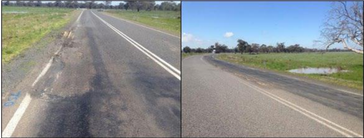
Images (above): Constraint 21.2 Federation - Pavement failure. Image from Federation Council
