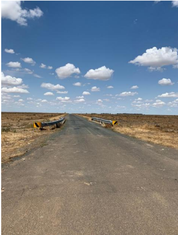
Image above: Constraint 17.13 Hay - Chainage 20.7km Bridge 4.5m wide
