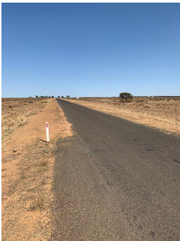
Image (Above) Constraint 25.4 Hay - Chainage 13.2km narrowing of the road to Chainage 28.1km from 8m to 6m
