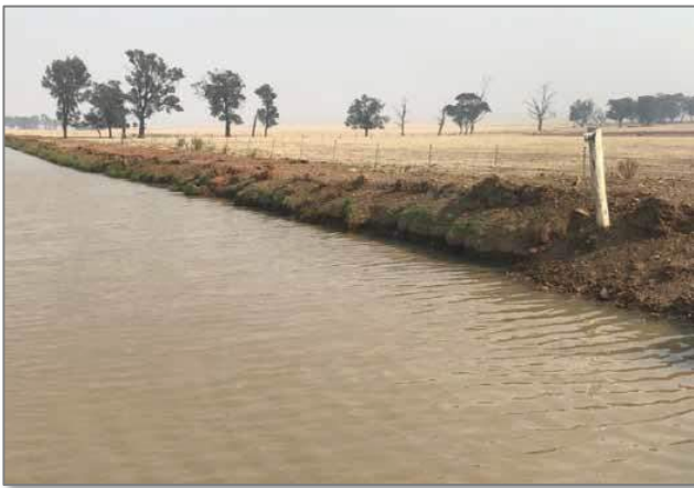
Mulwala Canal, December 2019. Photo commissioned by Berrigan Shire Council
