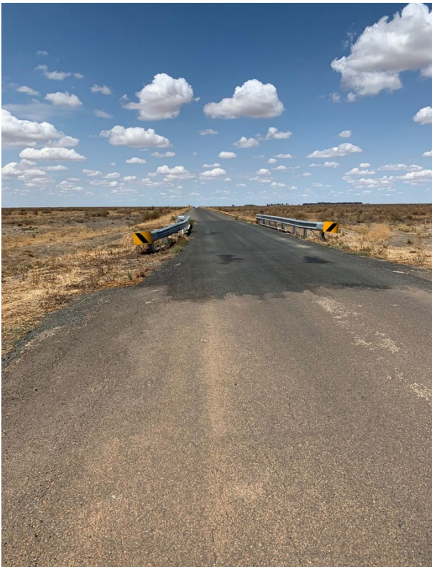
Image above: Constraint 17.9 Hay - Chainage 20.3km Bridge 4.5m wide
