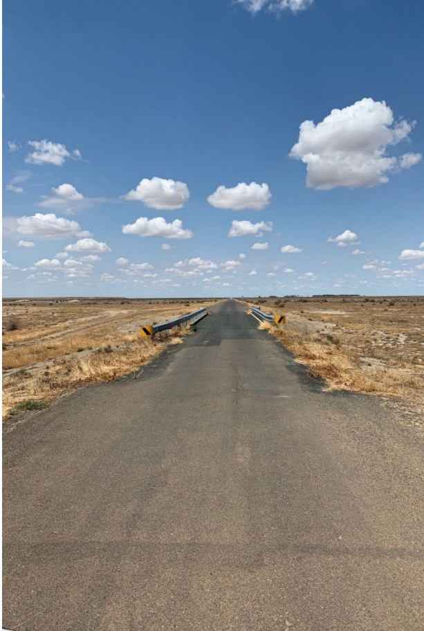
Image above: Constraint 17.8 Hay - Chainage 19km Bridge 4.5m wide
