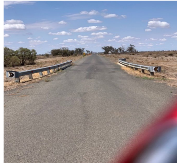
Images above: Constraint 17.7 Hay - Chainage 10.3 to 11.6km there are 6 x Culverts 4.5m wide
